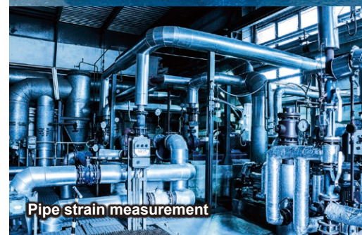
Brake and pipe strain measurement
